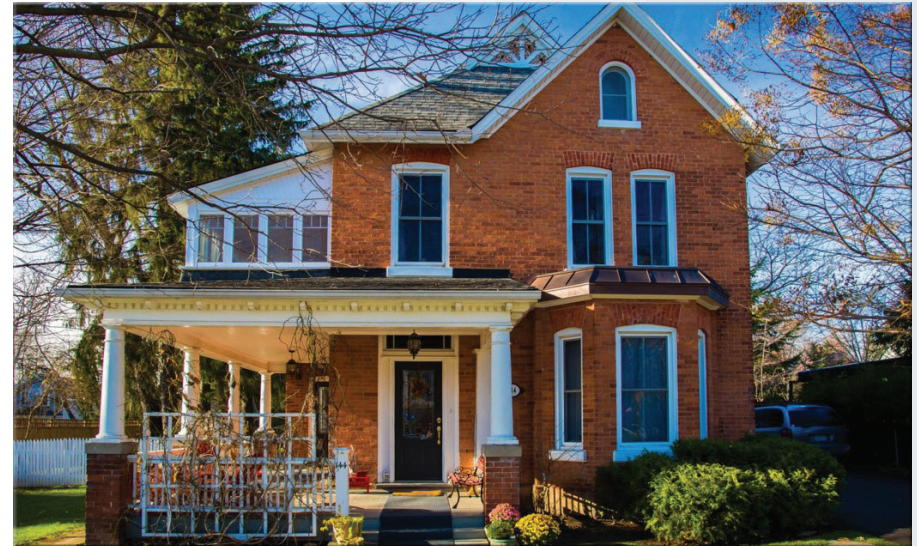
144 Maple Avenue (Heritage Property)
